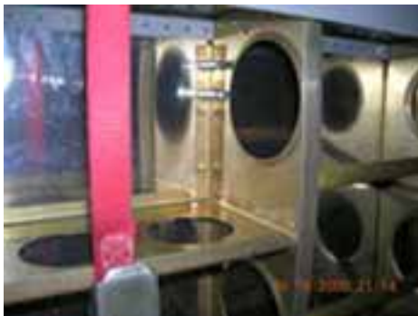
Sta. 20.0 Rib and bulkhead
